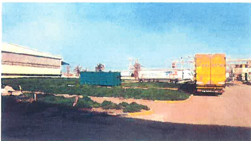
UF01 location – Urea finishing section and electrical substation
