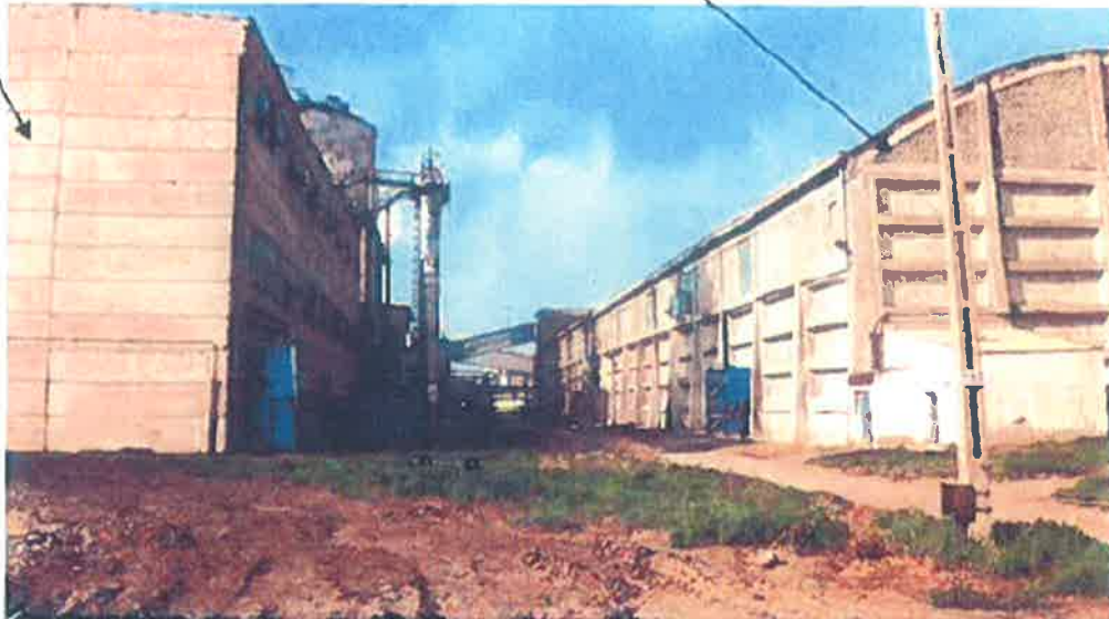
US01 location – Compressor hall and electrical substation
